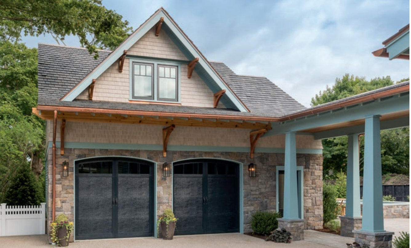
York Limestone with a dry-stack grout technique. Photo Credit: Nat Rea
